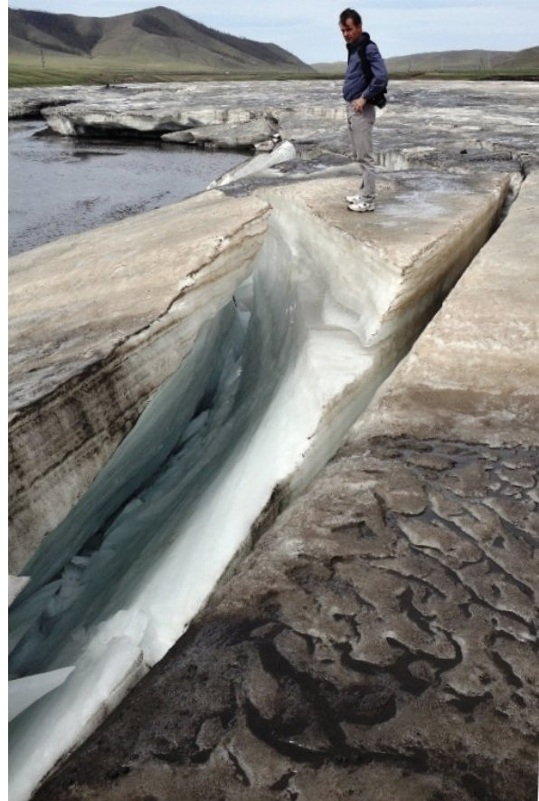
Figure 4. disintegrating naled ice shield in summer Structural failure of a naled ice shield in summer due to enlargement of a phreatic tube leading to collapse of the tube. (photo: Jim Reichert, World Bank)
